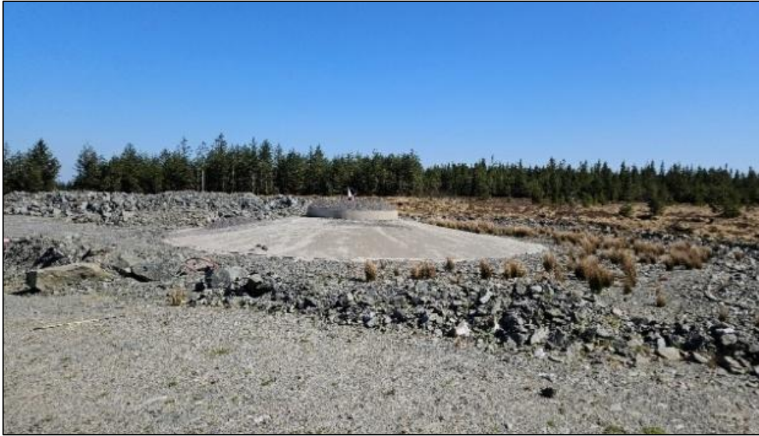
Plate 4-3 Predominantly finished turbine base with only backfill outstanding
