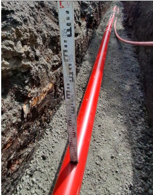
Plate 4-7 Typical Single Cable Trench View
