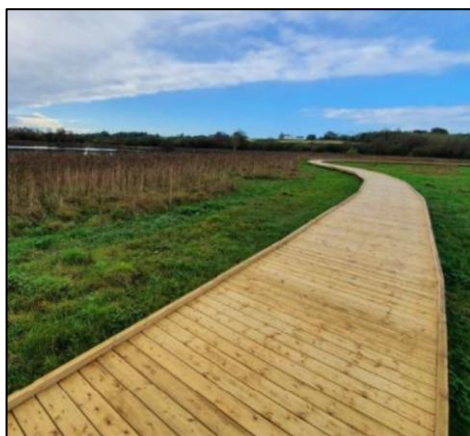
Plate 4-4 Typical completed boardwalk
