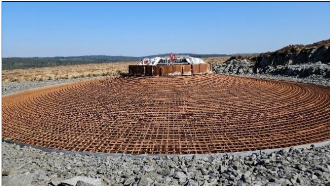
Plate 4-2 Turbine 'Anchor Cage'
