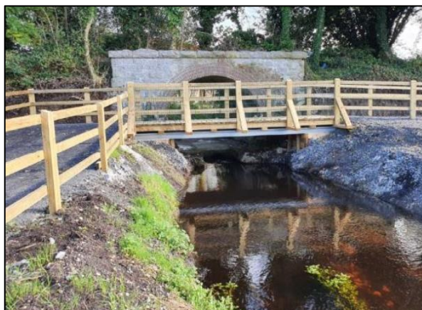
Plate 4-5 Typical bridge structure
