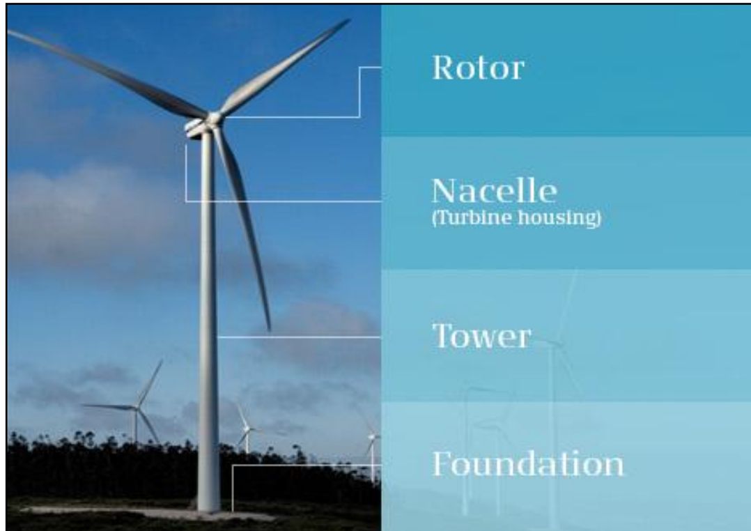
Plate 4-1 Wind turbine components
